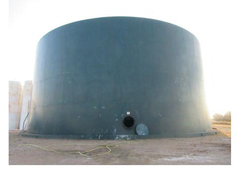
Tank # 1 West 73' Diameter X 32' High Tank Carbon Steel Construction 32% Nitrogen Solution
